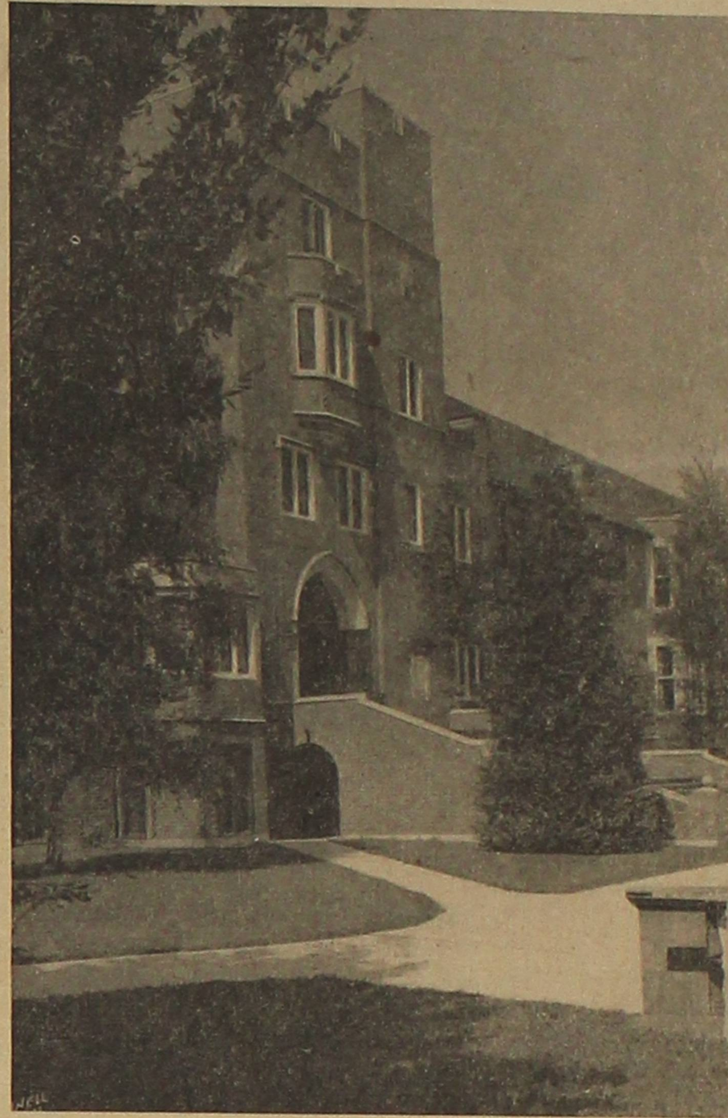
C. H. Jones Hall occupies the east side of the academic quadrangle. This building is the gracious gift of the late Mrs. Franke M. Jones in memory of her husband. It is a three-story structure of concrete and brick, 270 by 59 feet. The ground floor contains the library, alumni and field offices, YMCA and YWCA rooms, student and social rooms, and student offices. The first floor is occupied by the auditorium which seats over 700 people, the offices of the president, dean, bursar and registrar, and eight classrooms. The second floor is occupied by the balcony of the auditorium, ten classrooms, the small chapel and the faculty offices. The roof is decked and the attic is lighted by skylights. The art room and galleries are located here.
