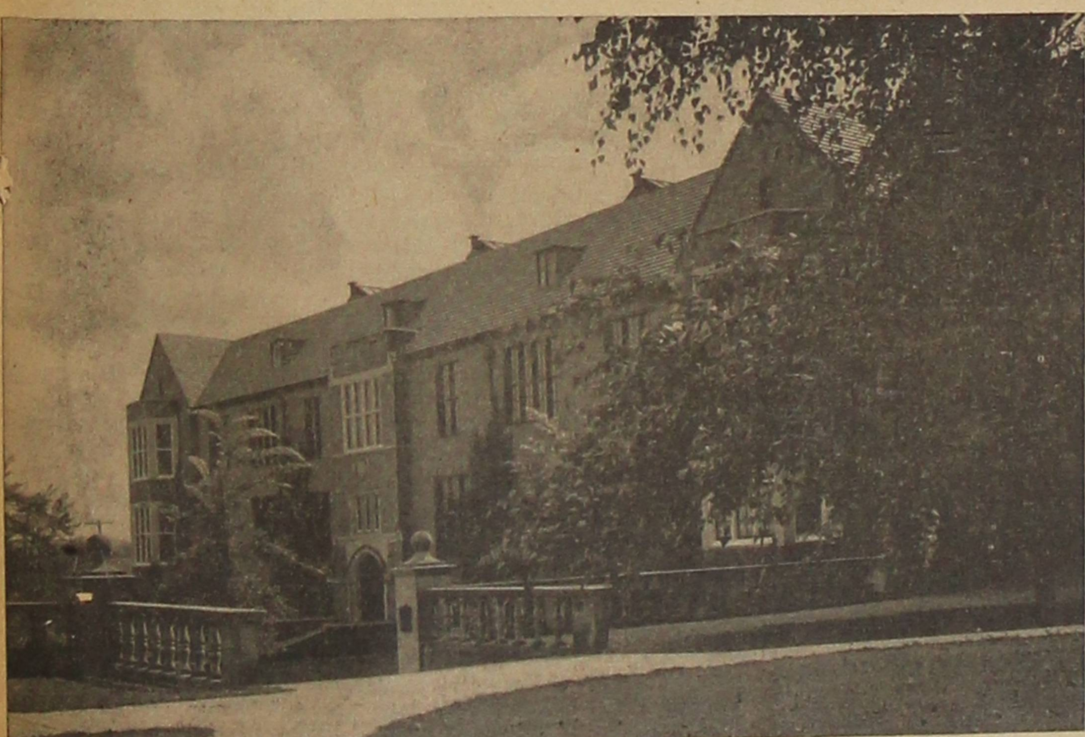
Leonard Howarth Hall of Science, completed in 1927, is a modern fireproof, three-story building of concrete and brick, 150 by 60 feet. The lower floor is occupied by the physical laboratories, the commons and the heating plant. The second floor houses the biological and home economics laboratories and class rooms. The third floor is occupied exclusively by the chemical laboratories, classrooms, and a modern lecture room. The attic, lighted by skylights, is used by the geology department for its classrooms and laboratories and by the Museum of Natural History.
